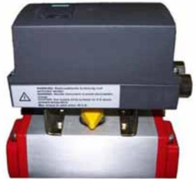
**Step 6:** Insert the pneumatic fittings on the positioner and actuator, run tubing from the outputs of the positioner to the inputs of the actuator.
